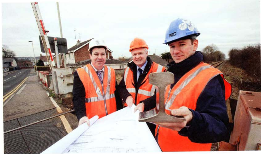
During March contractors BAM and FP McCann completed a £1.3m re-railing and drainage project on the 10 km Coleraine – Portrush branch, which has seen a 40% growth in passenger traffic since 2002.
